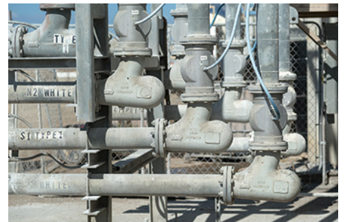
At this concrete production plant, the compact dimensions of the tight-radius Smart Elbow design minimize space requirements compared to long-sweep elbows.
