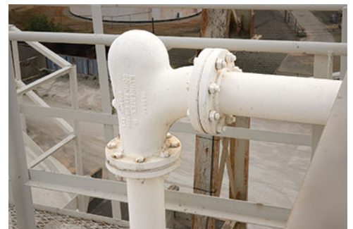
The Smart Elbow® deflection elbow installed in ready-mix plants prevents abrasive materials from impacting the elbow wall, eliminating worn elbows, related downtime and recurring maintenance costs.
