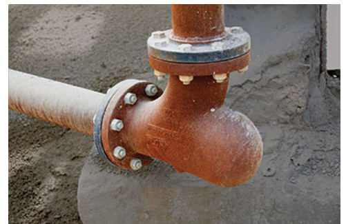
HammerTek short radius deflection elbows eliminated the need to weld or replace failed sweep elbows 100 ft in the air.
