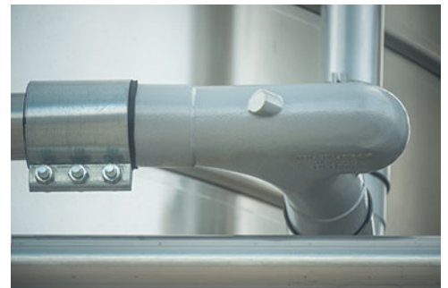
Smart Elbow® deflection elbows replaced conventional sweep elbows, reducing maintenance cost and downtime.
