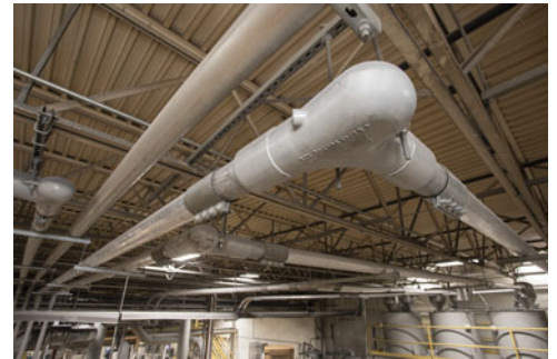
Smart® Elbow 90° deflection elbows prevent abrasive glass-fiber reinforced pellets from damaging pellets as well as blowouts at pneumatic line bends.
