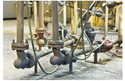
Waupaca Foundry deploys Smart Elbow® deflection elbows to avoid leaks, blowouts and downtime from wear by abrasive materials speeding through the pneumatic lines.
