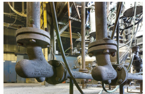
A spherical vortex chamber protruding from the elbow diverts part of the flow where it forms a loosely packed mass that slowly rotates in the direction of flow, gently deflecting particles around the bend.
