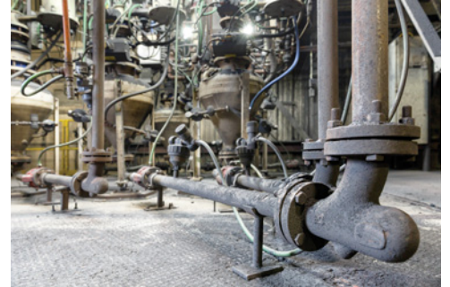
Waupaca Foundry deploys Smart Elbow® deflection elbows to avoid leaks, blowouts and downtime from wear by abrasive materials speeding through the pneumatic lines.
