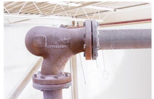
Installing short-radius deflection elbows put an end to leaks, spills, replacements and associated costs encountered with other type elbows.
