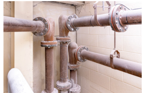
Installing short-radius deflection elbows put an end to leaks, spills, replacements and associated costs encountered with other type elbows.
