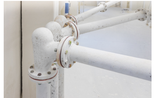
The Upper Occoquan Water Reclamation plant has gone 16 years without an elbow failure after installing short radius Smart Elbow® deflection elbows.
