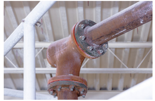
The Smart Elbow® deflection elbow features a spherical chamber in which incoming particles swirl in a slowly rotating ball, gently deflecting incoming material around the bend without impacting or abrading the elbow wall.
