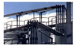
RheTech found that HammerTek Smart Elbow® deflection elbows could convey highly abrasive finished product with few signs of wear after a year in service. The sweeps previously used lasted only three or four months.
