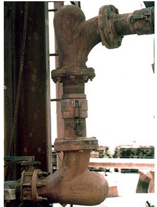
One of the new elbows installed at Chromalloy.
