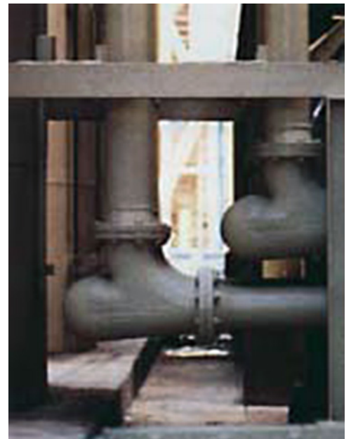
The compact design of the Smart Elbow deflection elbows saves space — the twelve 6in. elbows shown here occupy the same space as a large desktop. They may also be rotated on their flanges for greater design flexibility and installation ease.
