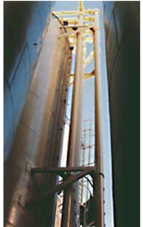
These 95' pipes were assembled on the ground and then stepped into their racks, greatly reducing costly crane time.
