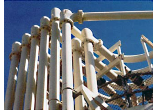
The compact design of the Smart Elbow deflection elbows saves space — the twelve 6in. elbows shown here occupy the same space as a large desktop. They may also be rotated on their flanges for greater design flexibility and installation ease.
