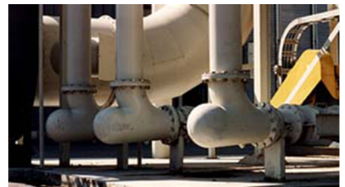
10 in. Vortex Vortex Ell elbows in new high pressure system.
