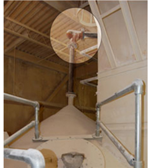
This 90-degree Smart Elbow deflection elbow from HammerTek, Bethlehem, Pa., diverts the pebble lime in the pneumatic conveying line into a silo for storage. The sharp turn that had tormented many different types of elbows has not been a concern for the Smart Elbow deflection elbow, nor for facility management.
