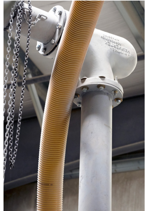
Smart Elbow® deflection elbows replaced European cast iron deflection elbows and sweep elbows with rubber inserts that failed at numerous bends.
