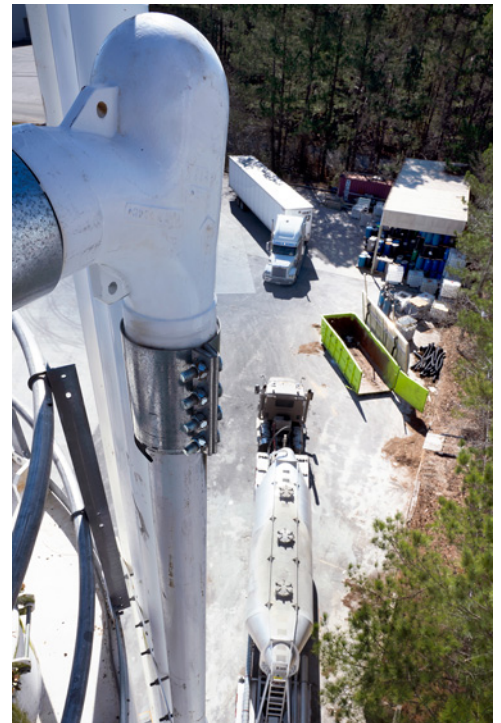
Fast-moving sand, conveyed from bulk trucks to silos, caused previous elbows to fail, prompting replacements with Smart Elbow® deflection elbows shown.
