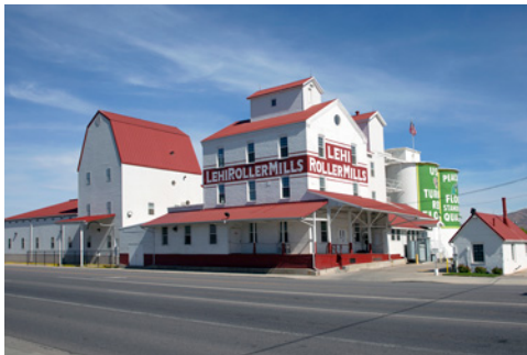
Founded in 1906, Lehi Mills processes 45 tons (49.6 tonnes) of flour per day in its original building.
