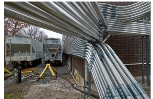
Approximately 123 million pounds (55.8 million kg) of PE is unloaded from railcars annually through pneumatic lines equipped with Smart Elbow® deflection elbows.
