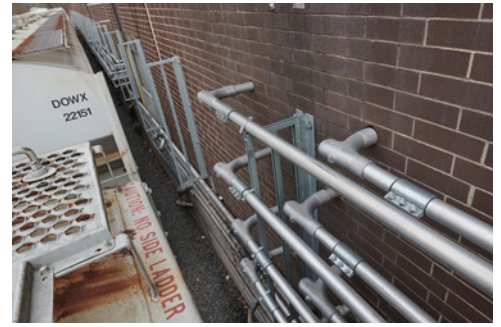
Smart Elbow® deflection elbows route material from rail cars to silos, and in turn, into the plant.
