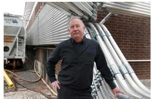
Ed Komoroski doubled the number of silos and added multiple pneumatic conveying lines at All American Poly's Piscataway, NJ plant.
